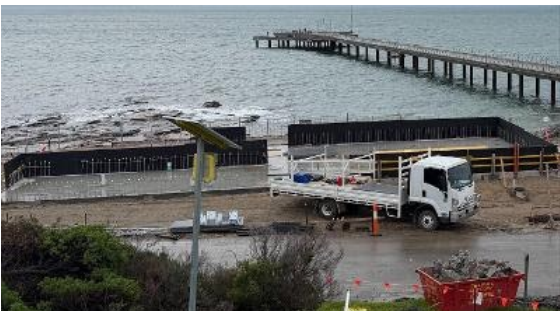
This is the start of the formwork around the perimeter of our slab to form the 500mm high concrete wall.
