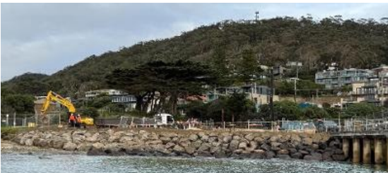
This is the completed sea wall South of the Pier. We were originally told that it was going all the way to our boat channel access ramp but if they had done that, and with the angle they have built the wall at, we would have lost a heap of boat trailer parking. It will be interesting to see how the exposed dirt bank in the gap survives. I reckon it will need a vertical rock or concrete wall there in the future.
