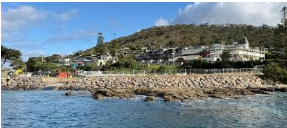
This is the finished wall on the town side of the pier. Our clubhouse is smack bang in the centre of it. Still in the world's best location.
