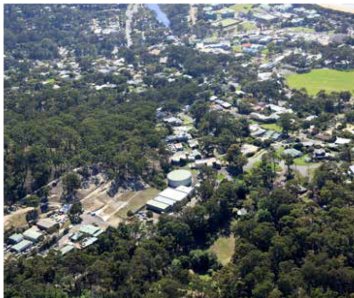
Lorne Water Treatment plant
